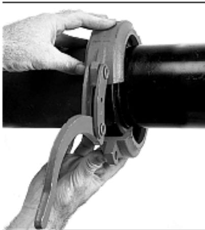
**4 HOUSINGS**— Put one half of the open coupling over the gasket as the coupling keys fit firmly into the grooves on each pipe end. Swing the other half of the coupling into position around the gasket and into the grooves.
