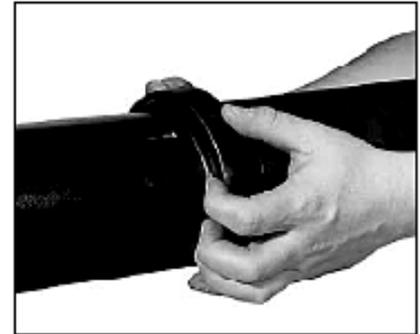
**3 ALIGNMENT**— After aligning the two pipe ends together, pull the gasket into position, centering it between the grooves on each pipe. Gasket should not extend into the groove on either pipe.
