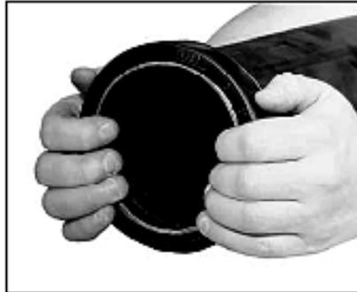
**2 GASKET INSTALLATION**— Slip the gasket over the pipe end making sure the gasket lip does not overhang the pipe end.
