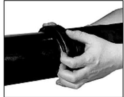
**3 ALIGNMENT**— After aligning the two pipe ends, pull the gasket into position centering it between the grooves on each pipe. Gasket should not extend into the groove on either pipe.
