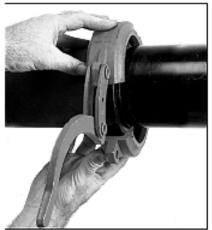
HOUSINGS— Put one half of the open coupling over the gasket as the coupling keys fit firmly into the grooveson each pipe and. Swing the other half of the coupling into position around the gasket and into the grooves.
