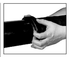
ALIGNMENT— After aligning the two pipe ends, pull the gasket into position centering it between the grooves on each pipe. Gasket should not extend into the groove on either pipe.
