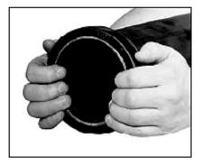
2 GASKET INSTALLATION— Slip the gaske: over the ploe end, making sure the gasket lip does not overhang the pipe end.
