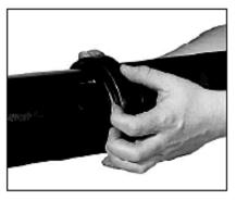
3 ALIGNMENT— After aligning the two plpe ends together, pull the gasket into position, centering it between the grooves on each pipe. Gasket should not extend into the groove on either pipe.
