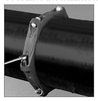
The instructions are based on pipe grooved in accordance with Gruvlok® grooving specifications. Check pipe ends for proper groove dimensions and to assure that the pipe ends are free of indentations and projections which would prevent proper sealing.
