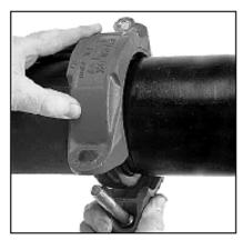
4HOUSINGS—With one nut unthreaded to the end of the bolt, unthread the other nut completely and swing the coupling housing haves over the gasket, making sure the housing keys engage the grooves. Insert the bolt and turn the nuts finger tight.
