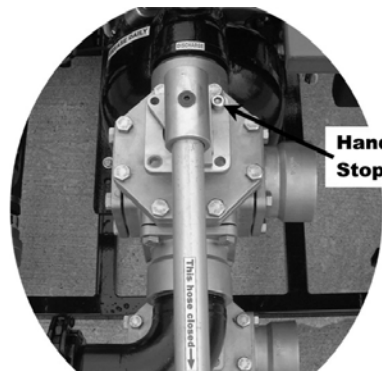
Valve Handles shown in the Cleaning/Treating Position
